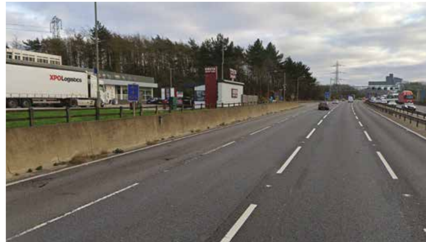
Figure 4 Toddington Motorway Service Area southbound merge showing concrete barrier © Google
