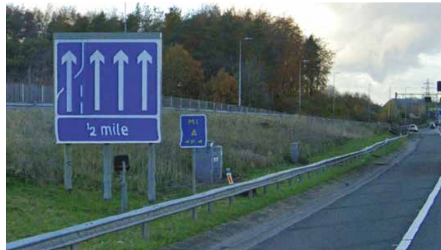
Figure 7 Verge FTMS showing the status of the downstream hard shoulder © Google
