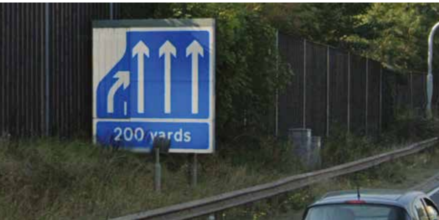
Figure 1 Verge sign showing the status of the downstream hard shoulder © Google
