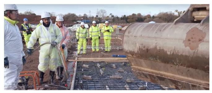
Trialling low carbon reinforced concrete on a temporary access road at junction 6 of the M42
