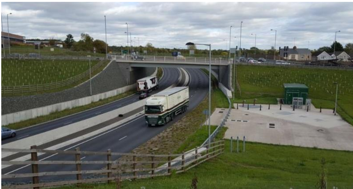
Figure 28: The pumping station on the south side of Tollbar End junction
