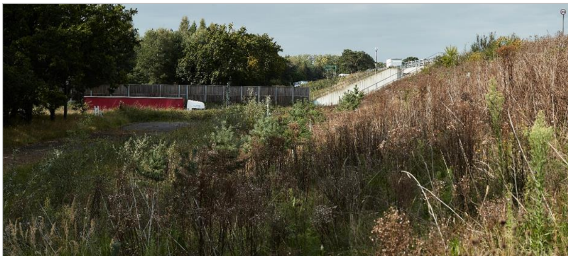
Figure 23 Planting plot on B1106 overbridge embankment at FYA
