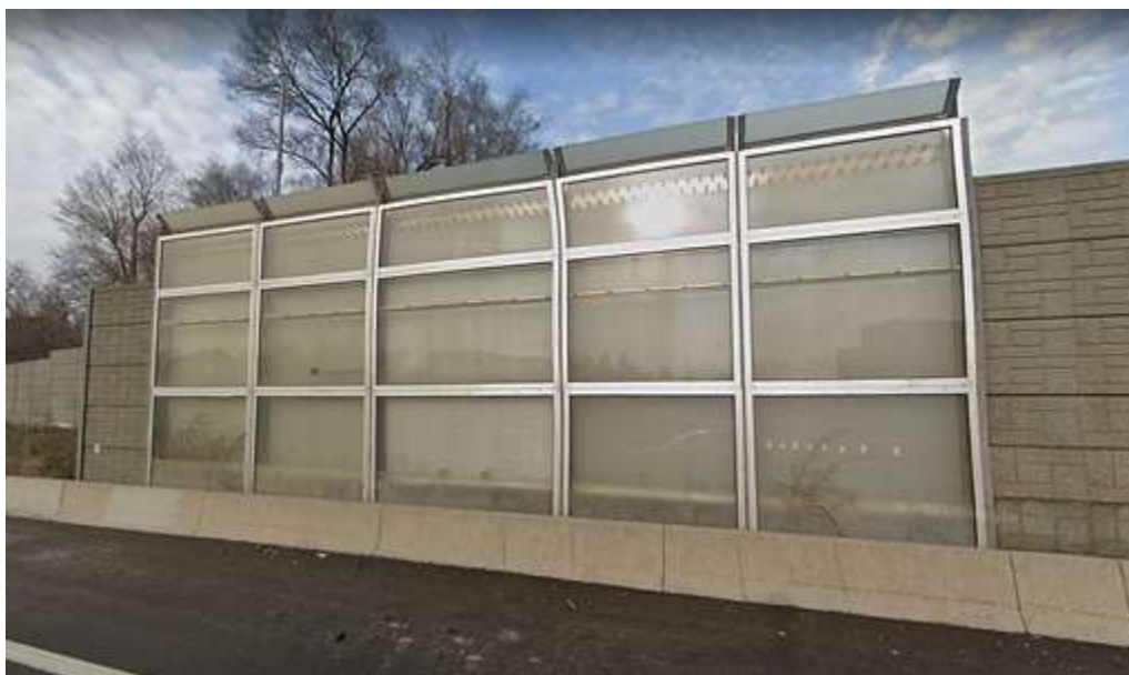
Figure A5: The SmogStop® barrier (15 m long and 6.5 m high; 5 panels installed) in Toronto, Canada at the intersection of Highway 401 and Bayview Avenue as part of a field trial. Image taken from Google maps.
