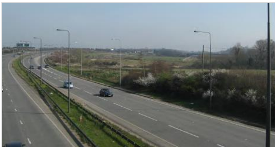
Figure 14 View from Ship Lane and local cycle route before the project
