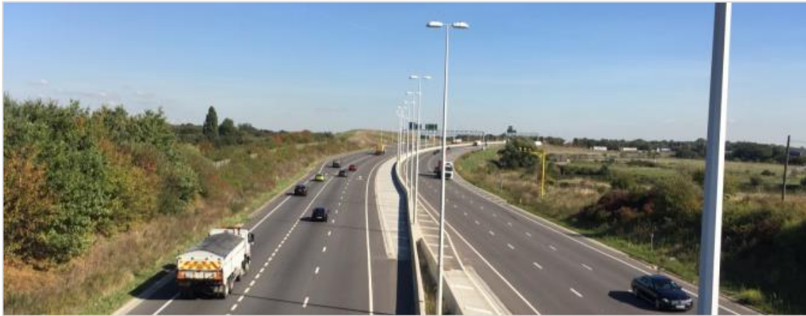
Figure 15 View at one year after looking east along A13 to M25 J30 from Ship Lane overbridge illustrating kerb edge drainage, hardened central reserve and upgraded lighting
